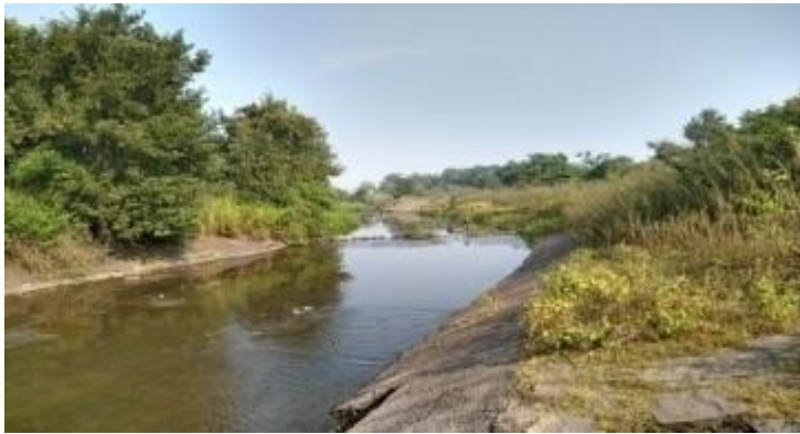
Stone embankment along Jamunia river
